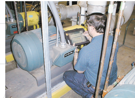
Dan Voss – Condition-Based Maintenance Motor Technician at Boeing – uses an electronic clipboard loaded with EM2 software to collect motor nameplate data during routine preventive maintenance. CBM staff entered over 180 of the larger motors in the plant in a matter of months.
