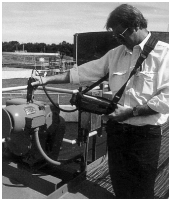
WI field consultant conducts an on-site vibration analysis of a clarifier pump motor.
